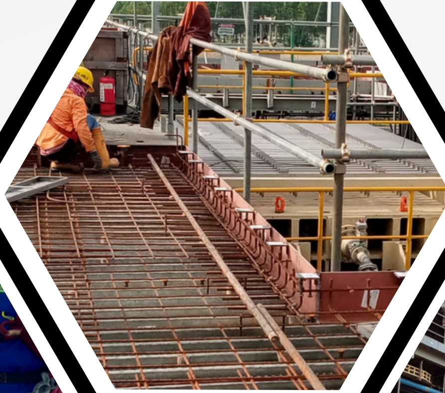
Rebar Installation
