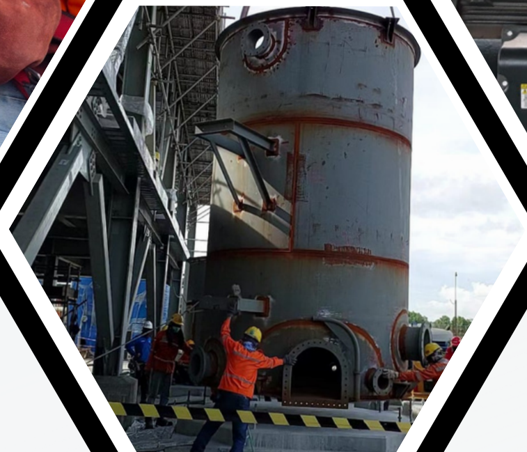
Tank Lift and Place
