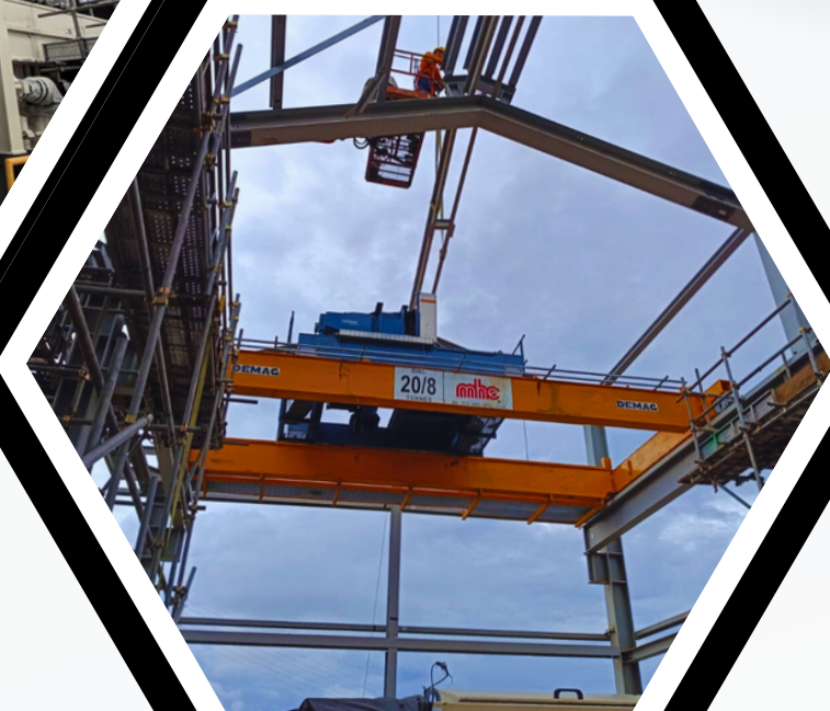
OHC Installation
