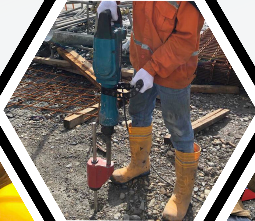
Ground Rod Installation
