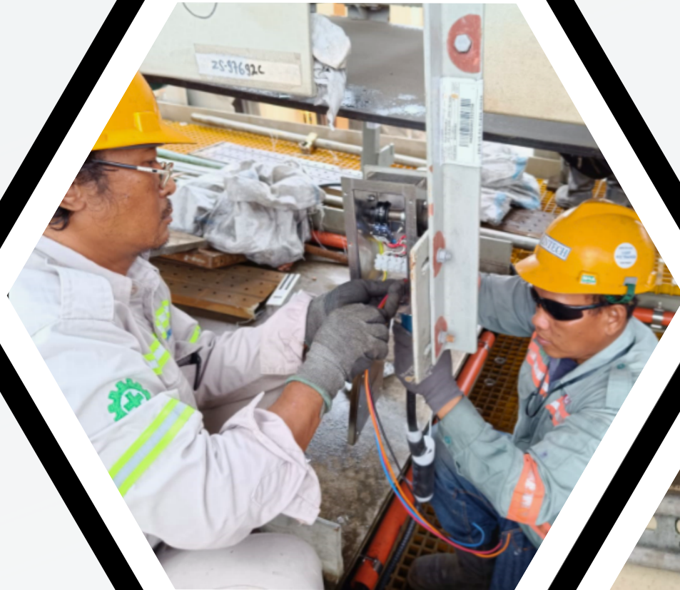
Belt Sway Indicator Installation
