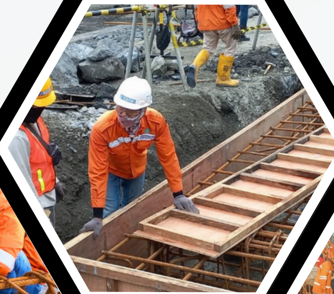
Formwork Installation
