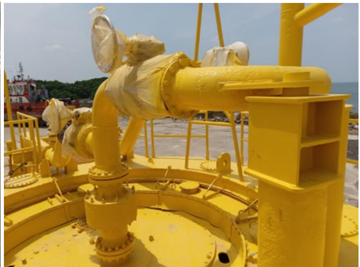
SPM SO1179 after repairs
